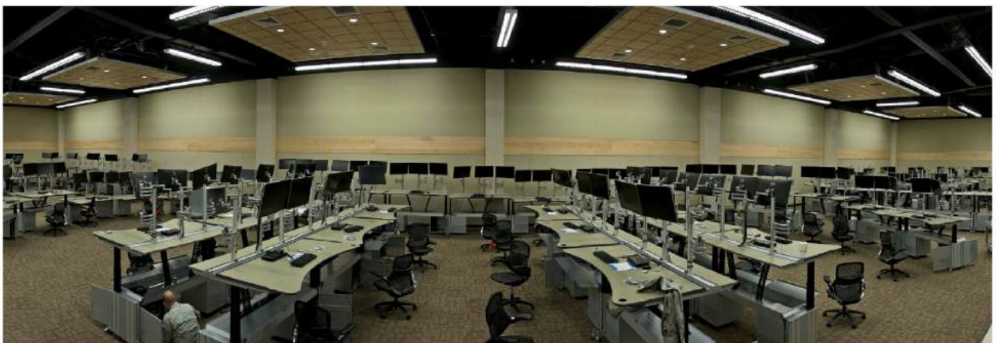
FIG/05 — OPERATIONS FLOOR FIT-OUT: CONSOLES, DISPLAYS & ENCLAVE CABLING
